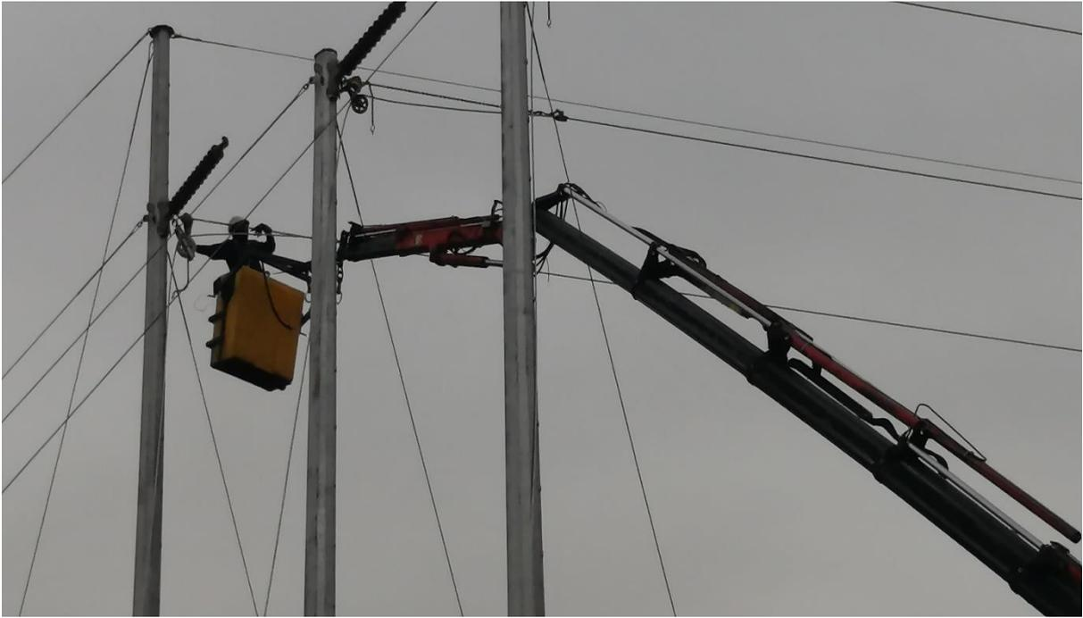
Figure 5: Tensioning of the electrical cables.
