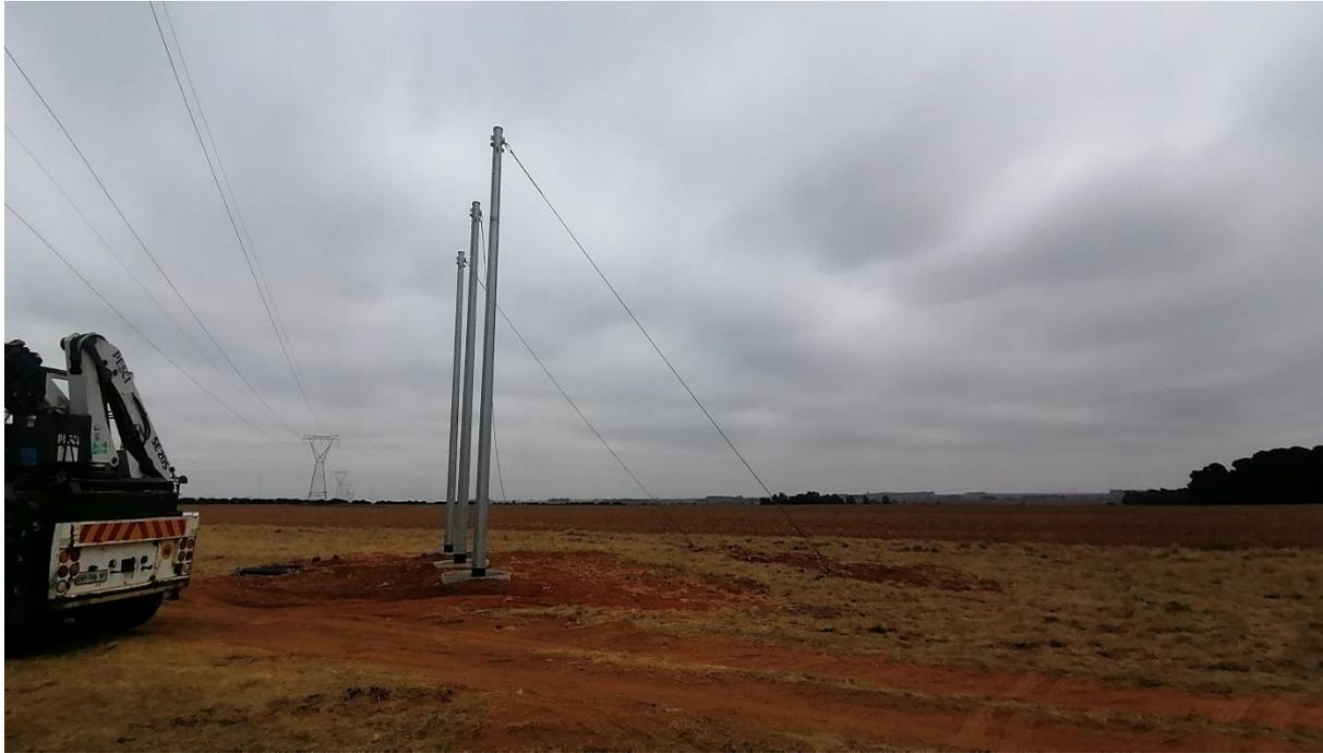
Figure 3: View of erected steel monopoles.
